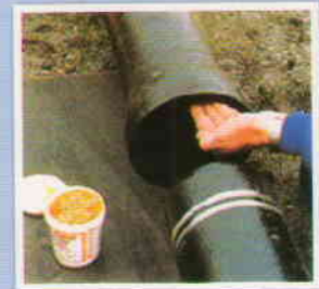
Apply lubricant onto the inside surface of gasket
