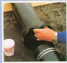
Insert the gasket into the socket
