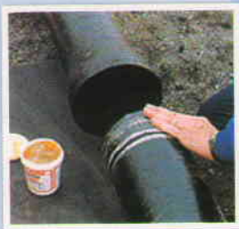
Apply lubricant to the spigot end
