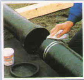
Clean the socket and spigot
