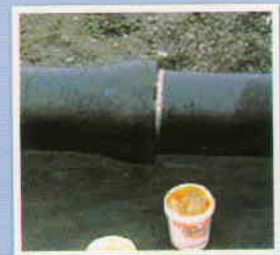
Guide the spigot into the socket & push
